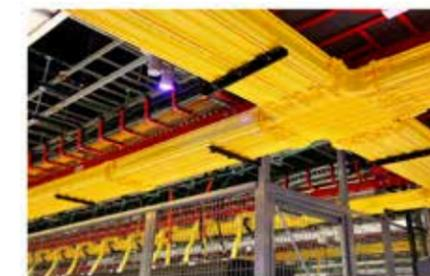
The Equinix cross-connect uses single-mode fiber (SMF) optic cables that run through a large, yellow overhead tray and down the aisles of the Equinix facility to the cloud peering switch in the AWS and Azure cages.
